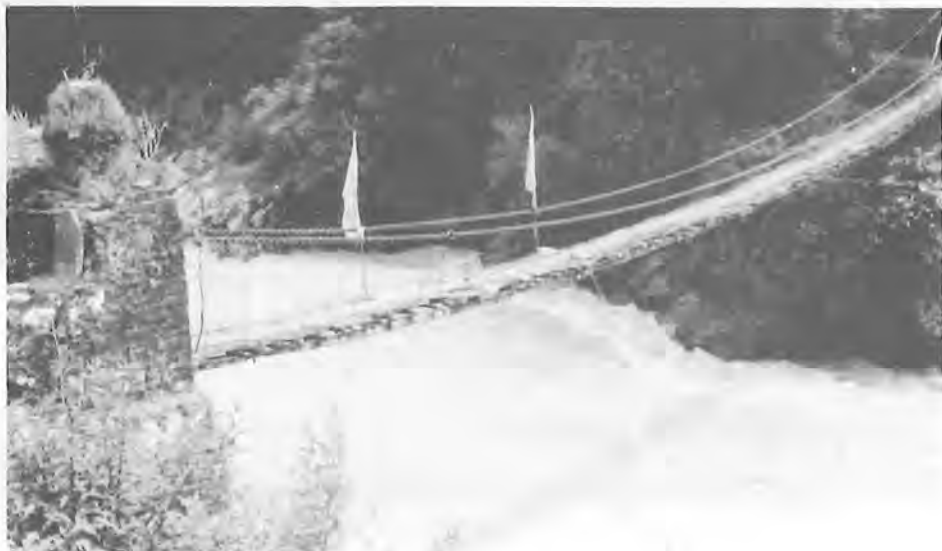
5. Permanent bridge over the Modi river.
