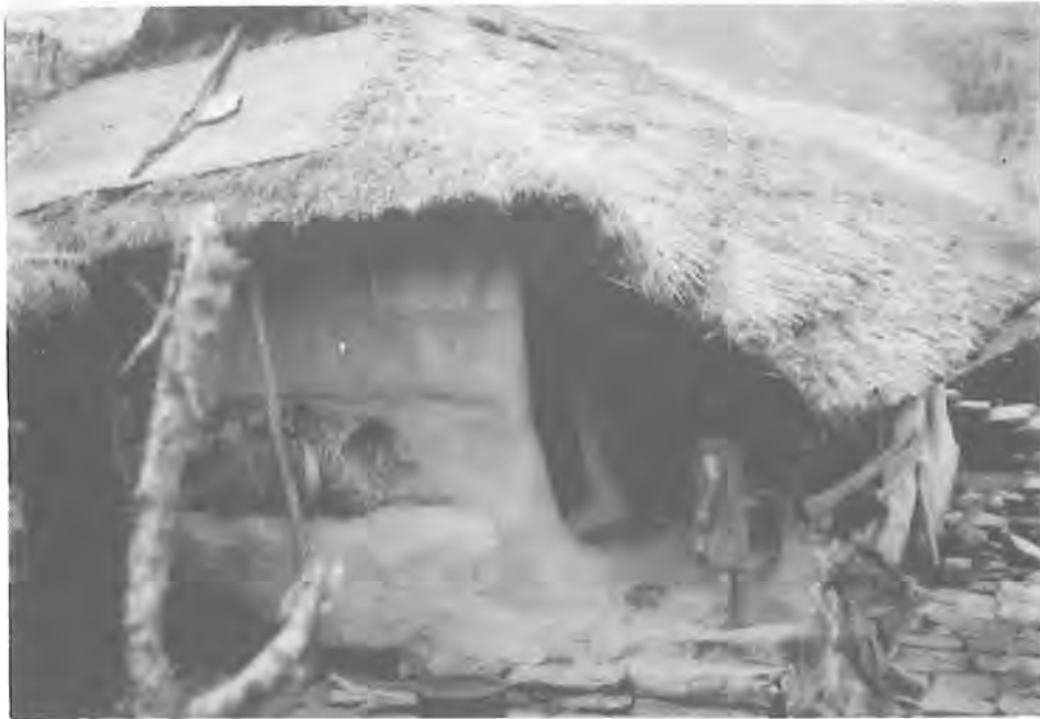
22. House N built of wooden planks covered with mud.
